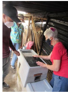
Onil stove installation
